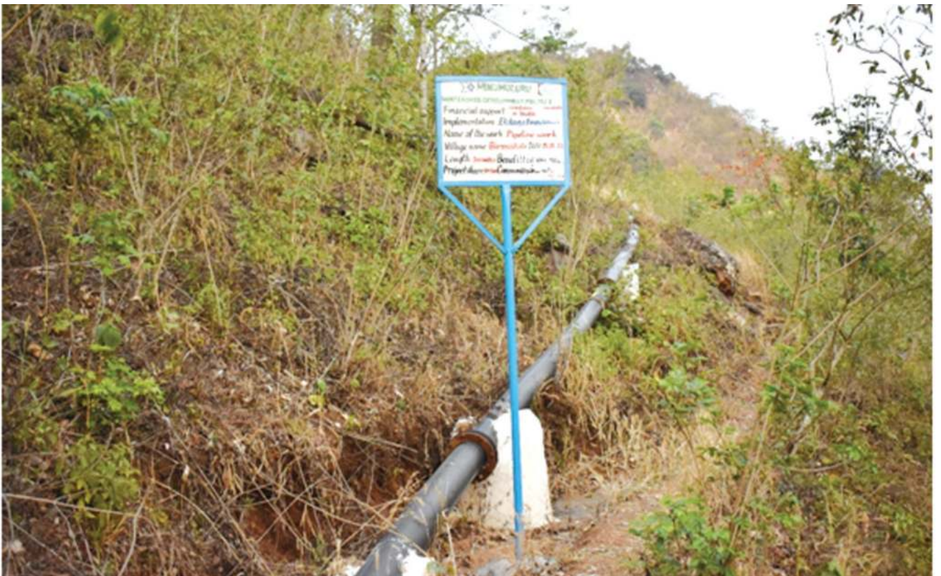
300 mtrs pipe line constructed
